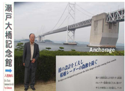
Fig.4 Bisan-Seto-Ohashi Bridge between Honshu and Shikoku
